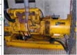
Exemple : diesel SDMO QAS 40 KD (32,9 kW / 40 kVA)
